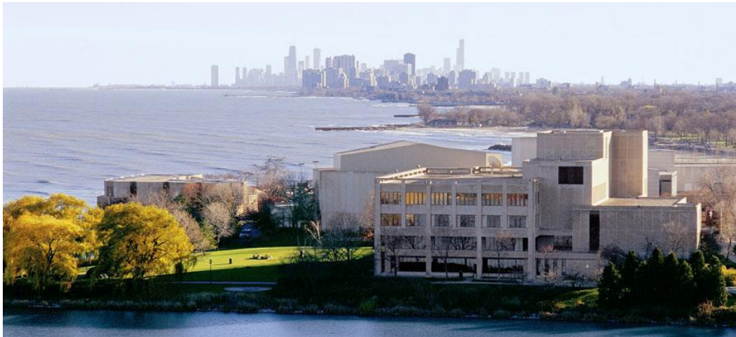
Northwestern University's Norris Center located on Lake Michigan
